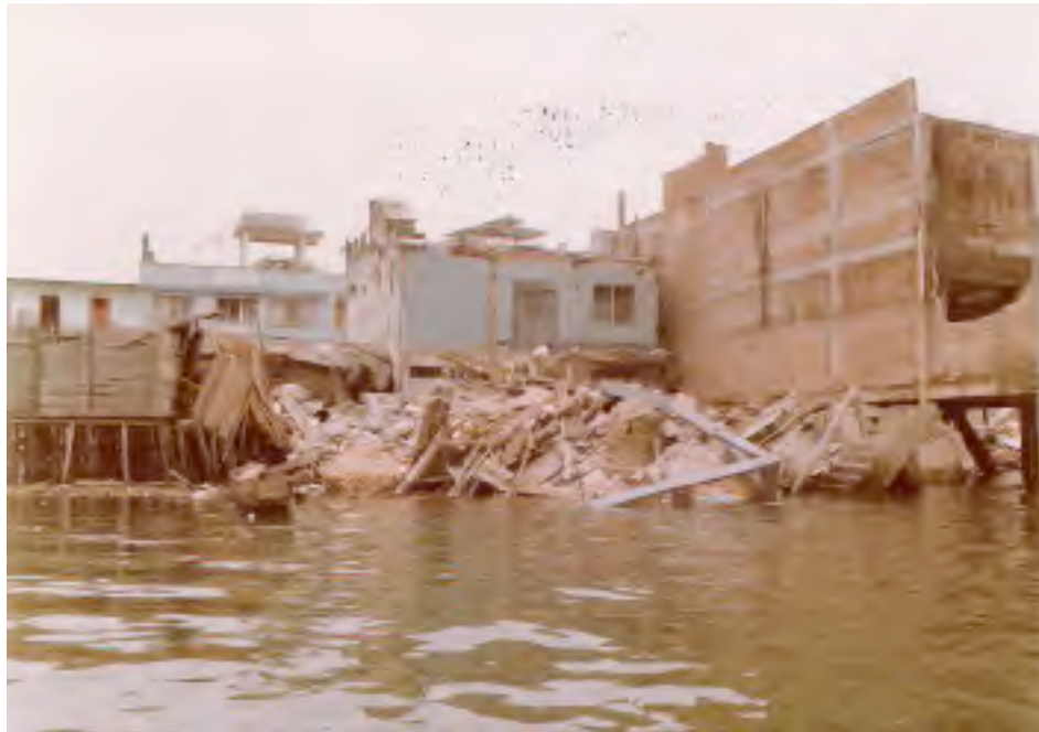
Figure 5. Tsunami damage at Tumaco (photo by G. Pararas-Carayannis)
